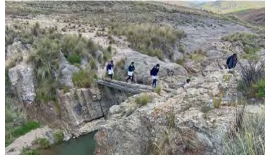
Makeshift Bridge Used by the Community of Tiraque, Bolivia to Cross the Suraj Mayu River
